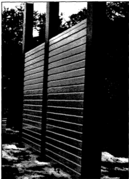
Close-up photo shows Carsonite panels installed between the flanges of the I-beam posts.
