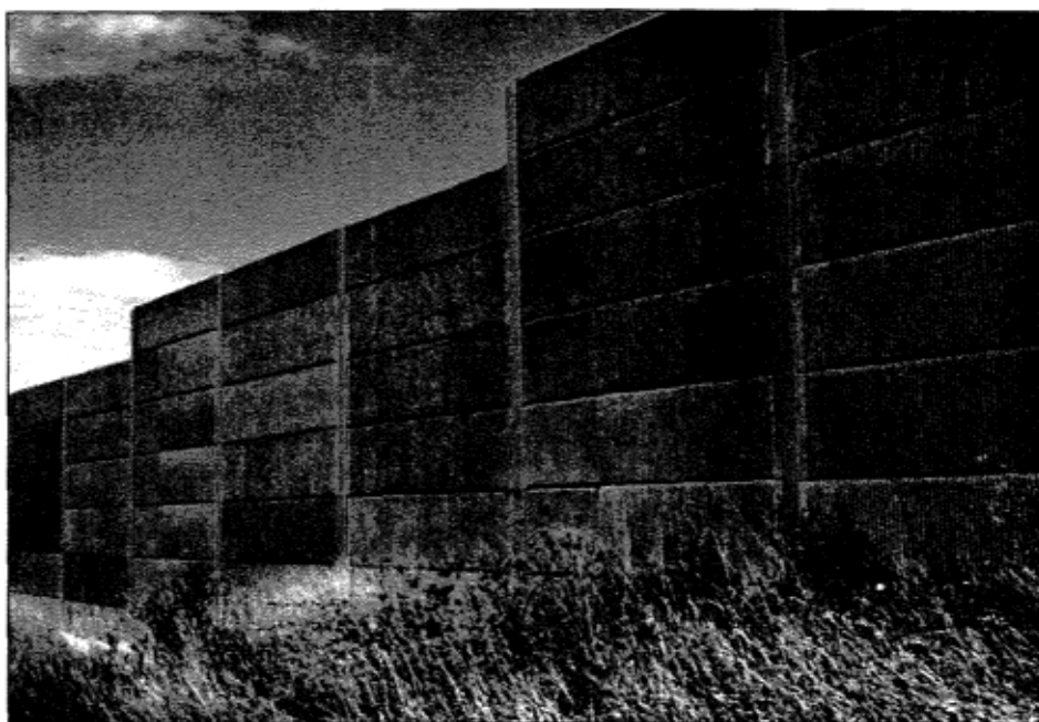
Spacing of the smooth-textured columns were coordinated with wall grade changes. Panel joints were aligned horizontally to create a neat and flowing appearance to the highway travelers and to the residential community.
