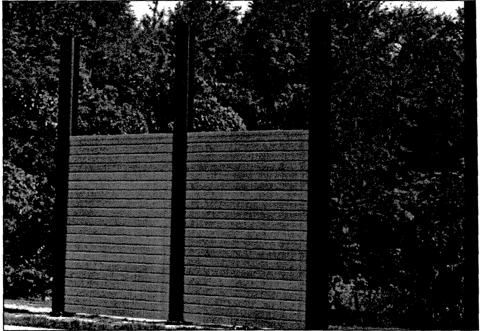
Photo of the Maryland SHA Demonstration/Display Facility, showing the pre-assembled Carsonite Sound Barrier panels installed in the I-beam posts. Locations of the poured concrete pile foundations for the posts are shown in the drawing below.
