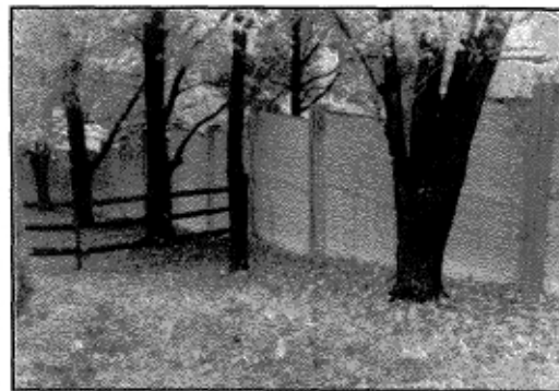
PLYWALL'S installation creates very little site disturbance. This barrier was installed a few months earlier with no damage to the trees or overhanging limbs. Sloping ground is easily accommodated.
