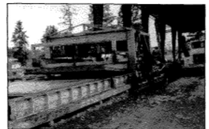
The IMPRESSOR — In actual production of wall panels for the above project
