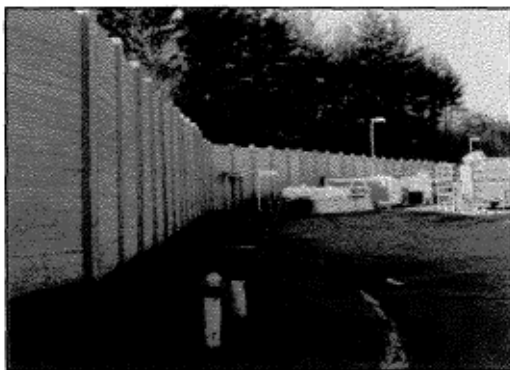
This bottling plant had received noise complaints from nearby homes. The complaints stopped after installation of this 15-foot high PLYWALL barrier.
