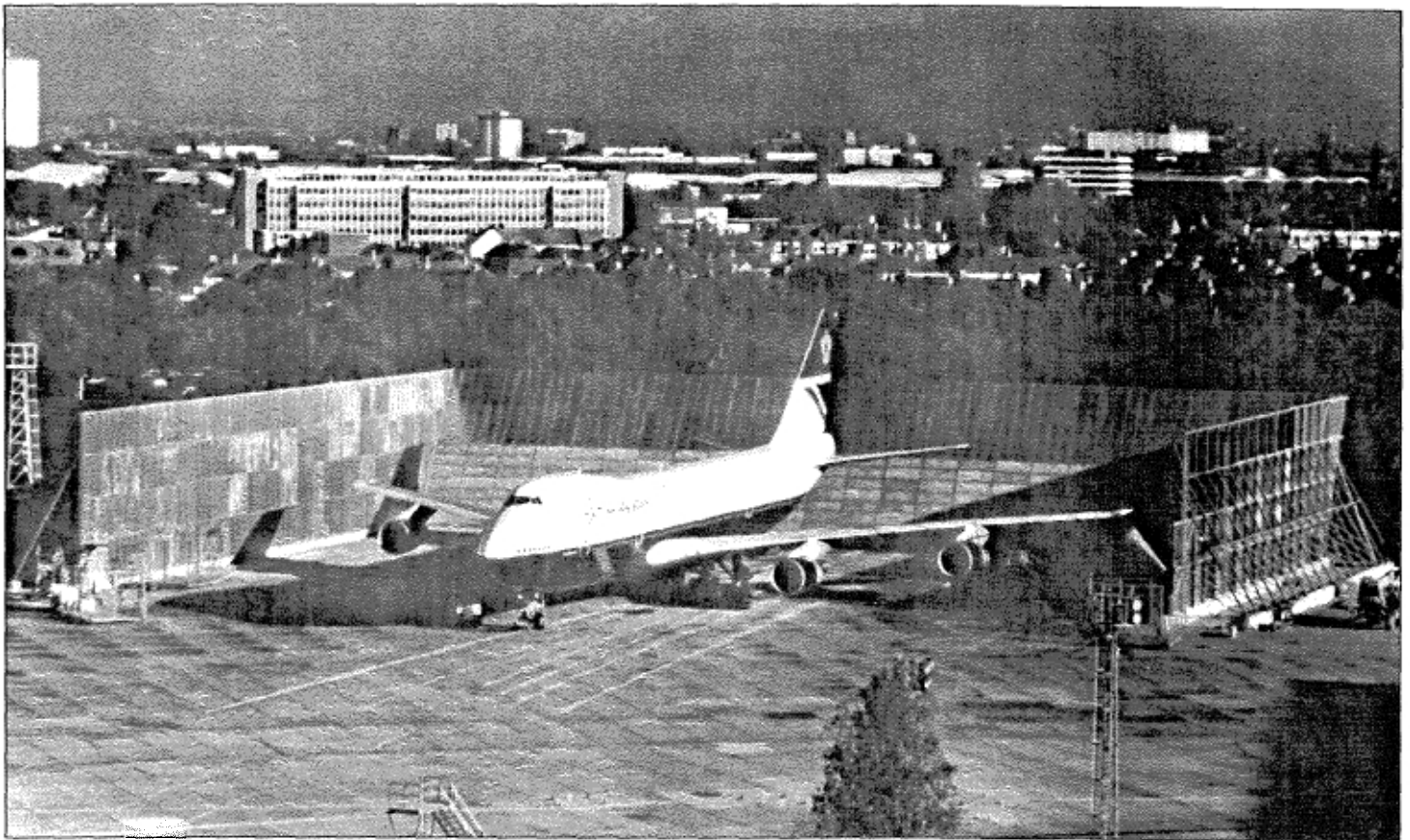
Ground Run-Up Pen reduces noise in residential communities bordering London's Heathrow Airport. Designed, built and installed by Industrial Acoustics Company, this type of acoustic structure can be used by airlines, airports, aircraft and aircraft-engine manufacturers to reduce noise to tolerable levels in communities neighboring their respective facilities.
