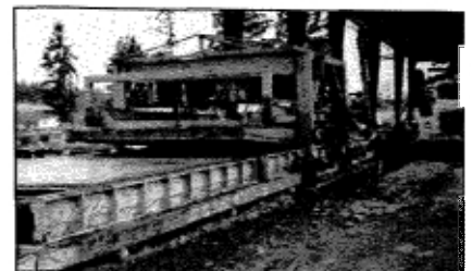
The IMPRESSOR — In actual production of wall panels for the above project
