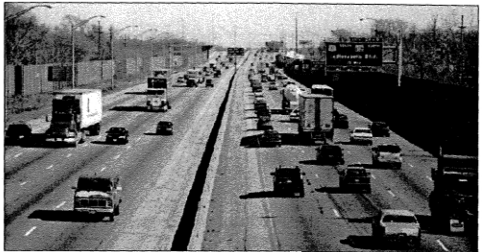
I-80/94 Borman Expressway carries 150,000 vehicles per day. Sound barrier design was modeled for 192,000 vehicles per day by the year 2016.
