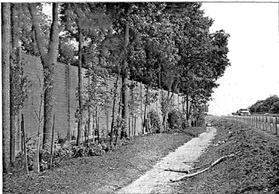
With the watchful eye of a full-time resident engineer, trees adjacent to the noise barrier were saved as well as the overhead canopy
