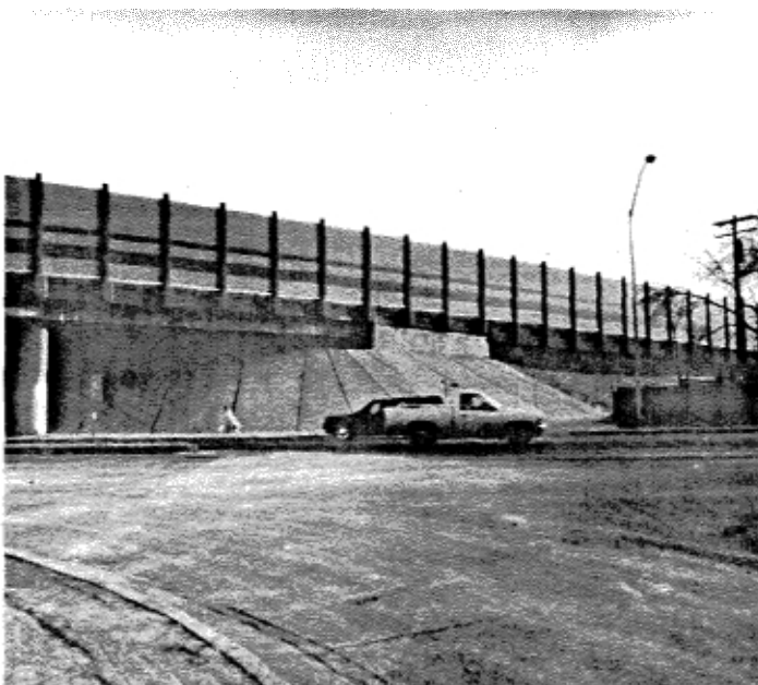
Photo features one of Carsonite's newest completed projects in Las Vegas, Nevada on I-15 southbound at the Sahara Blvd. exit.
