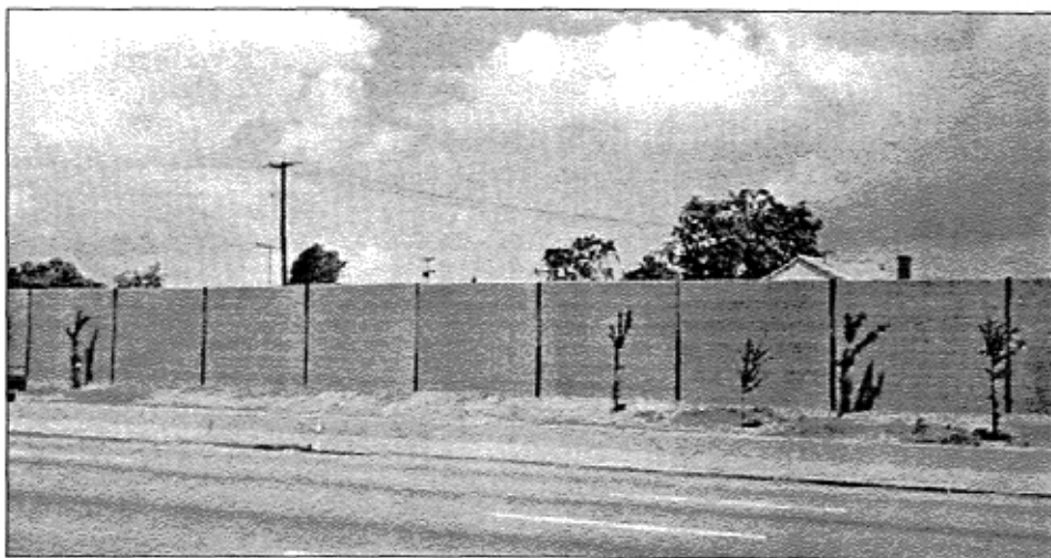
Highway view of Soundcore project in Cleveland, Ohio. Steel posts are spaced 24 feet on centers, and the 48"-wide panels are 'stacked' to the 24 foot height of the wall.
