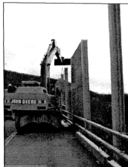
Flanged steel posts were installed with only minor reinforcement to the bridge.
