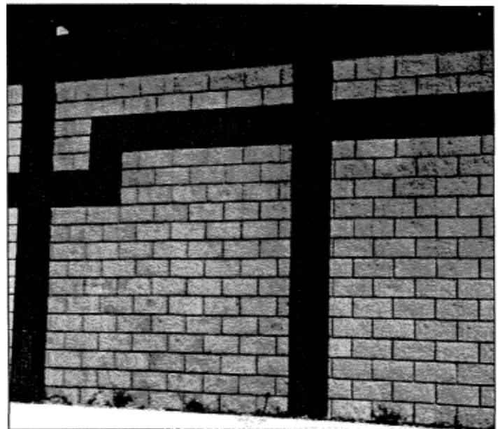
The ILong Island Expressway Coated with Cementrate WB Soundwall produced by Superior Precast
