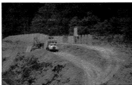
Noise Barriers being installed in the early phases of road construction. The hilly terrain is fairly typical of the area, which has affected construction cost.
